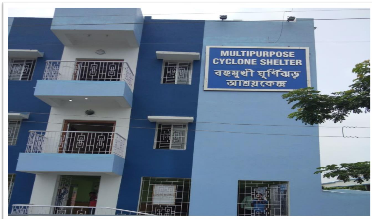
Uttar Mathbari Cyclone Shelter under Sandeshkhali-I Block under NCRMP – II
