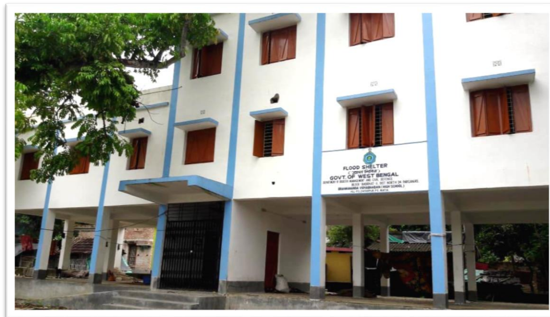
Flood Shelter at Brahmananda Vidya Bhaban under Bashirhat-II Block
