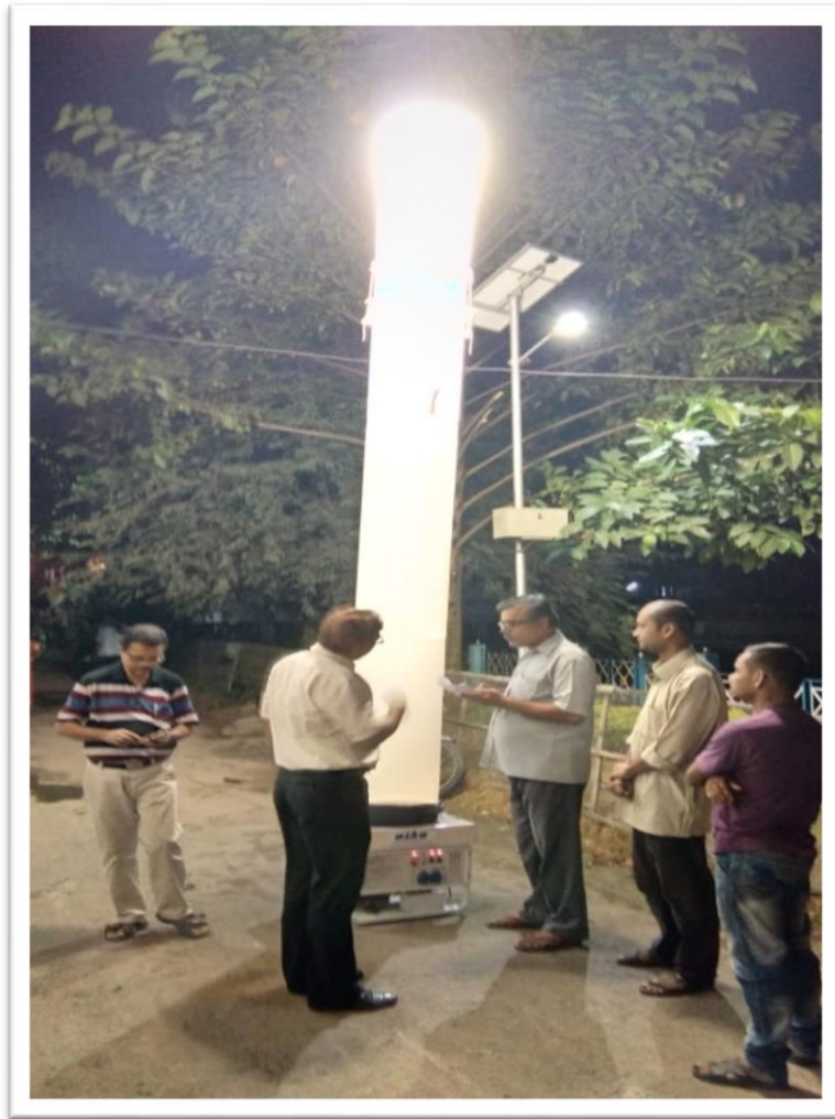
Dry run of tower light at District headquarters on 11.09.18
